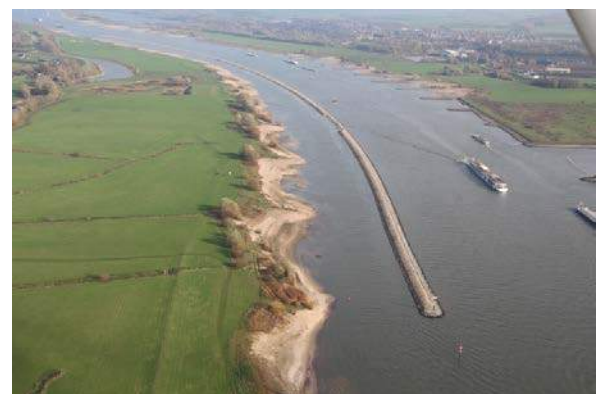
Figure 2. The LTD in the Waal River near Ophemert, looking upstream. Picture from Rijkswaterstaat Oost-Nederland.
