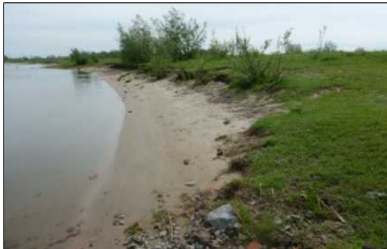
Figure 1. Nature-friendly bank at Welsumer Waarden in 2017, shortly after protection removal and excavation
