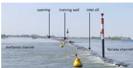
Figure 3. Inlet sill at upstream end of the longitudinal training wall at Wamel.
