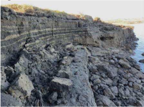
Figure 1. Eroding steep edge of the bank levee at Wamel with clear layering of more clayey and more sandy sediments.
