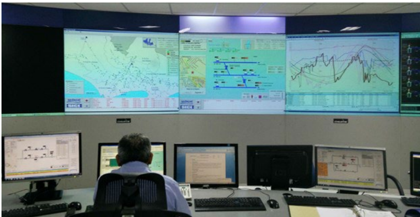
Figure 2.2 The central control room at the La Atarjea water treatment plant. Source: (IDOM, 2015).
