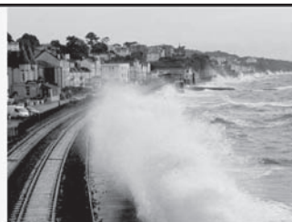
Hazards to railway
