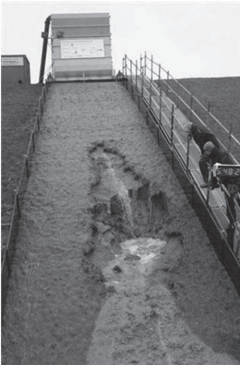
Figure 4. Damage to a dike section during a test with 75 l/s per m wave overtopping.
