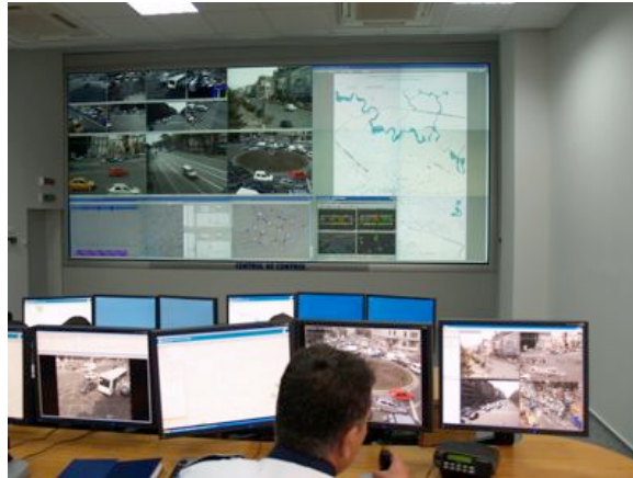
Figure 1.1: Traffic control room example.
