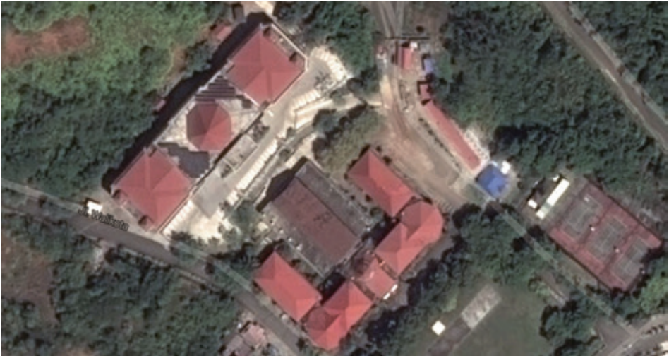
Fig. 5.2. Aerial view of the district office in Jayapura. Images ©2014 CNES / Astrium, Map data ©2014 Google.
