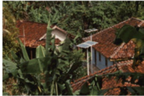
Fig. 1.1. Solar Home System in Sukatani, Indonesia [1].
