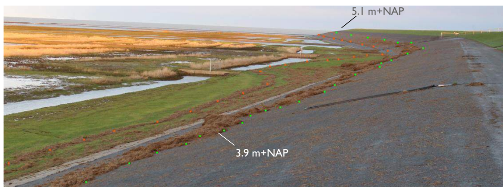
Figure 1: Two lines of flotsam ('veekranden') on the dike at the transition from a mudflat to a salt marsh
