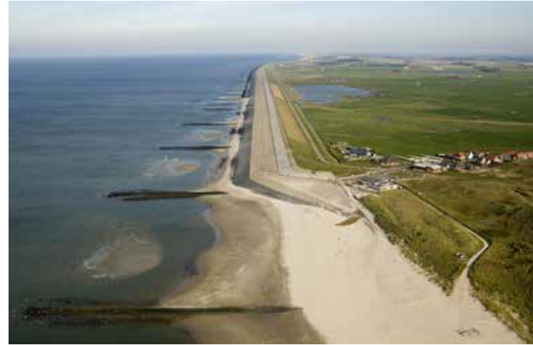
Figure 2a and 2b. (below) Illustration of "hard" versus "soft" engineering. The photo on the left shows the original "Hondsbossche en Pettemer Zeewering", a large dike in North Holland, whereas the photo on the right shows the same construction fortified by sand nourishment rather than additional hard structures. (Photo credit: Boskalis.)
