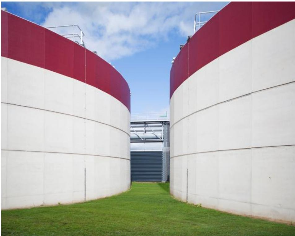
**Figure 2:** The first full scale Nereda plant (the plant consists of three basins in a parallel order)
