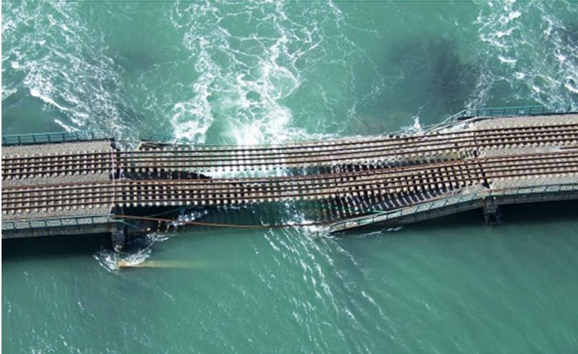
**Figure 1.** Malahide Bridge Collapse (21<sup>st</sup> of August 2009)
