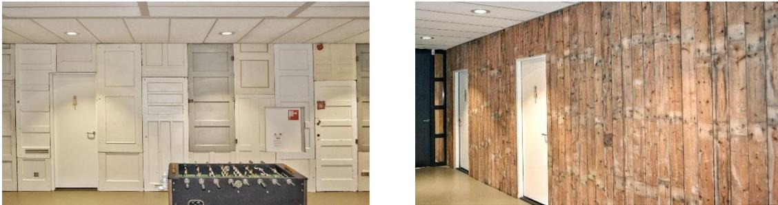
Fig. 2. Reuse of recovered doors (left) and floors (right) to decorate walls in a circular interior design project (Media Park)
