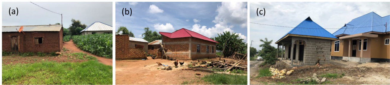
Fig. 1 Typical construction techniques in Tanzania. a Adobe dwelling; b rare burnt clay brick building with reinforced cement concrete (RCC) horizontal and vertical bands; c sand block building. Photograph by Giulia Jole Sechi, Iringa, Tanzania 2021
