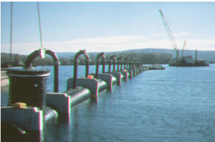
Figure 2: Diffuser configuration example (here floating before installation on the bottom). The risers are bended sideward and the ports are still closed.
