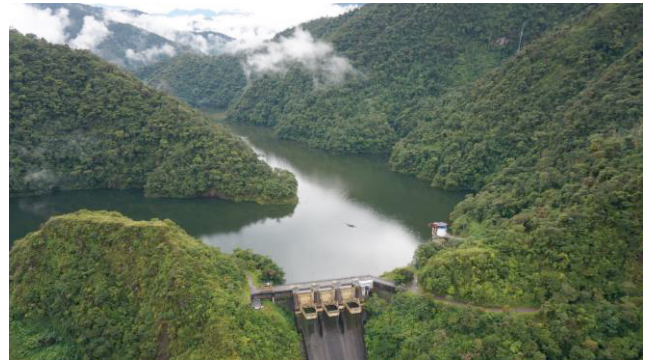
Fig. 1. Reservoir of the Alto Anchicayá HPP.
