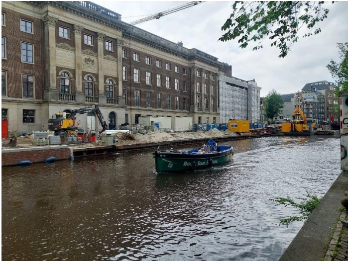
Fig. 3. Typical situation of a quay wall and pavement renewal
