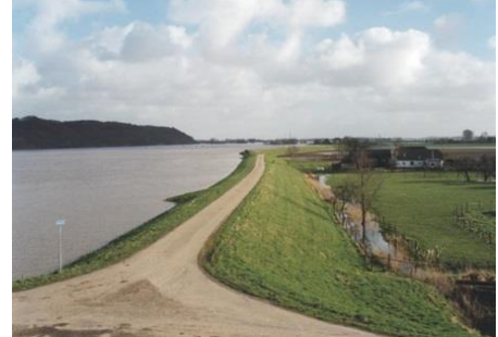
Figure 1.1. Dike with a road at the crest (Cormont, 1995)
