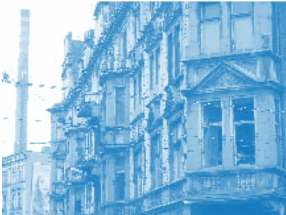
Inner-city residential building before demolition in Bytom (Photo: A. Haase)
