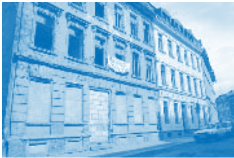
Old built-up stock in Leipzig / demolished building Leipzig-Plagwitz (Photo: A. Haase)
