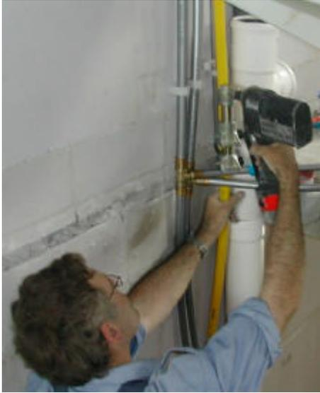
Figure 3: Even in difficult situations a press connection can be made in a few seconds
