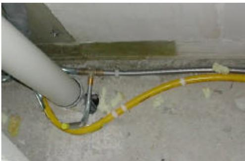
Figure 2: PEX pipe is very flexible and does not show load yielding. Complicated situations could be solved easily without using fittings.
