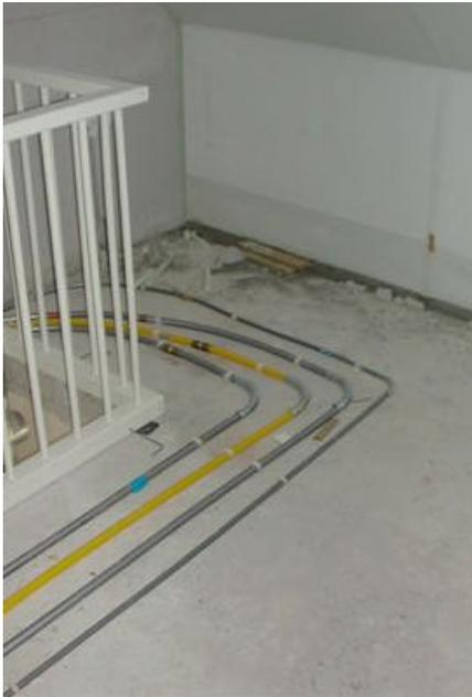
Figure 1: A yellow PEX pipe for gas amongst other PEX pipes. The pipes are now visible, but just hours later all pipes were covered by a layer of concrete. The time between laying and covering with concrete is as short as possible in order to prevent damage to the pipe work system.
