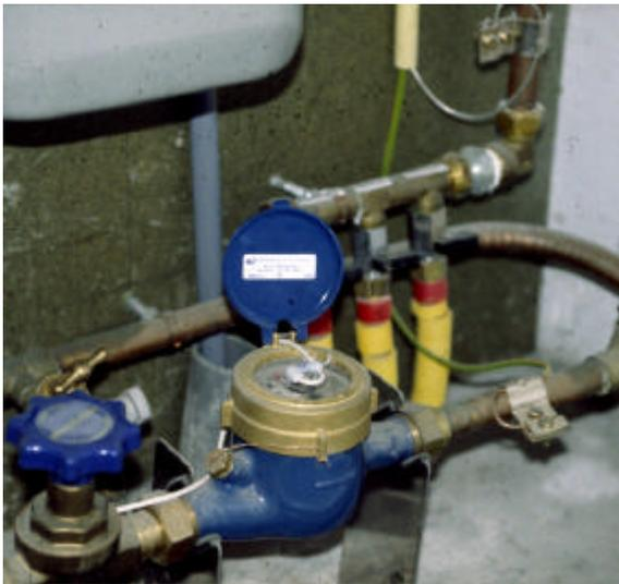
Figure 4: Short lengths of PEX pipe in the meter cupboard. The PEX pipes are protected by a corrugated plastic pipe. In this case a manifold has been applied. In the manifold, excess flow valves have been incorporated.
